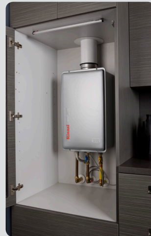
Example of an HDi200 internal installed in a cupboard - Rinnai Auckland showroom.
